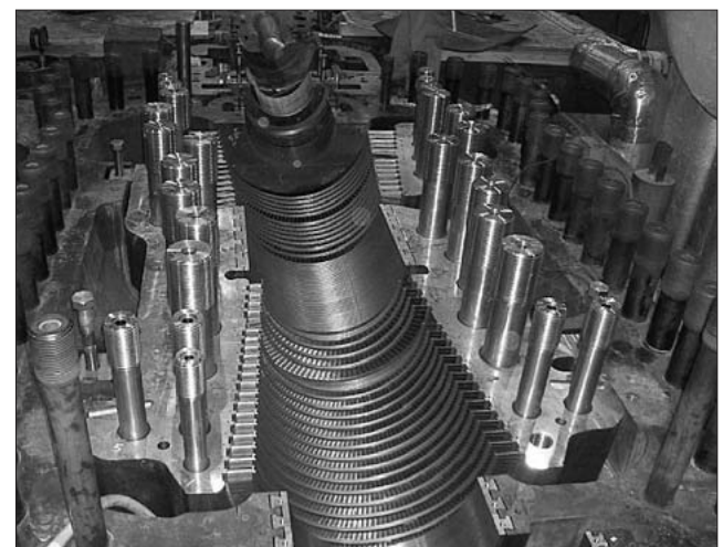
Fig.8 New high/intermediate pressure internal casing partially assembled onsite
