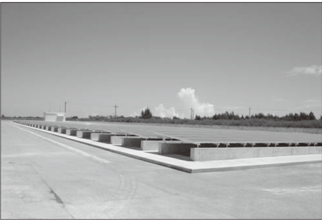
Fig.9 Overall view of system (Taramajima)
