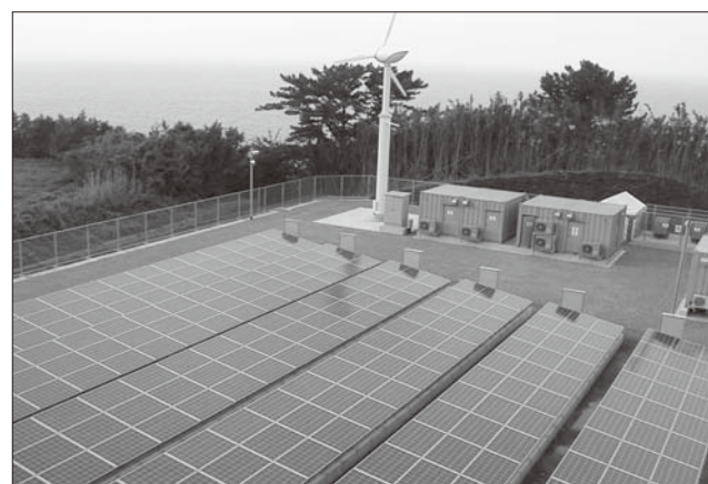
Fig.8 Overall view of system (Kuroshima)
