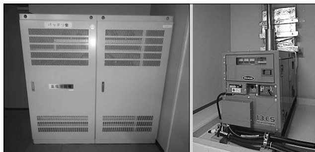
Fig.2 Installed state of backup power supply equipment
