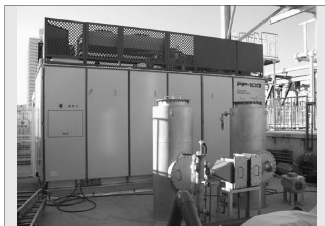
Fig.5 Fuel cell equipment under demonstration test
