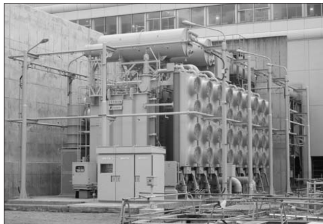
Fig.24 1,050 MVA main transformer
