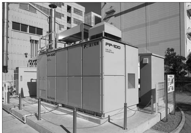
Fig.7 Fuel cell equipment installed in Kawasaki factory
