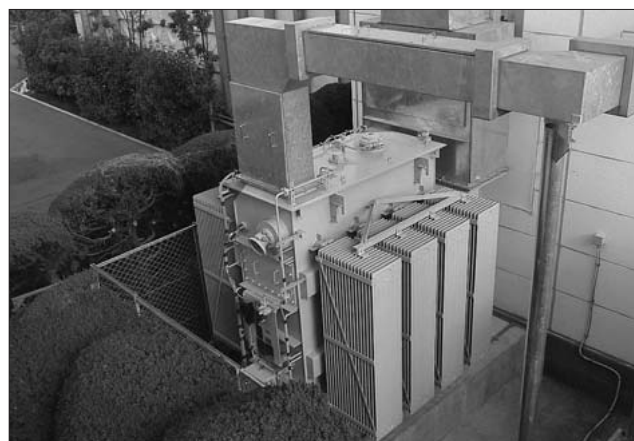
Fig.36 Ecore Trans (22 kV to 6,000 kVA)
