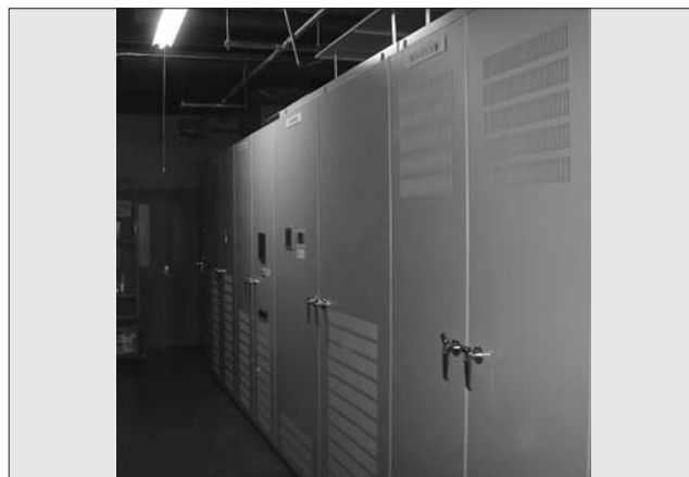
Fig.35 Medium-voltage UPS unit using lithium-ion capacitor
