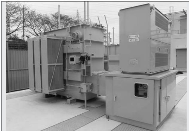
Fig.27 66 kV power-receiving and direct-current transforming facility
