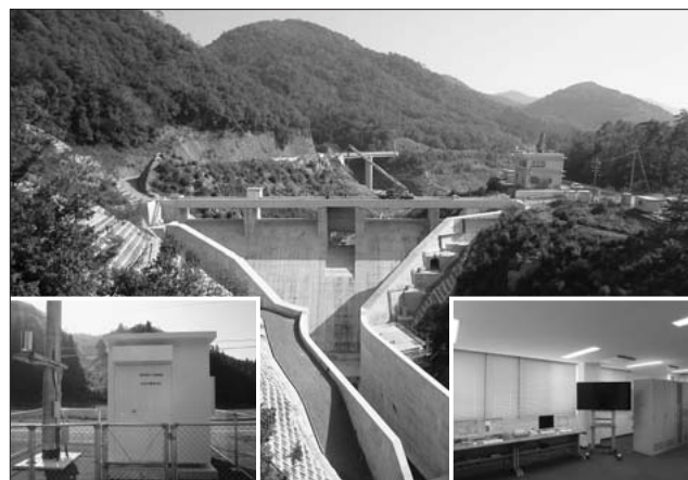
Fig.11 Telemeter and discharge warning equipment and dam control station
