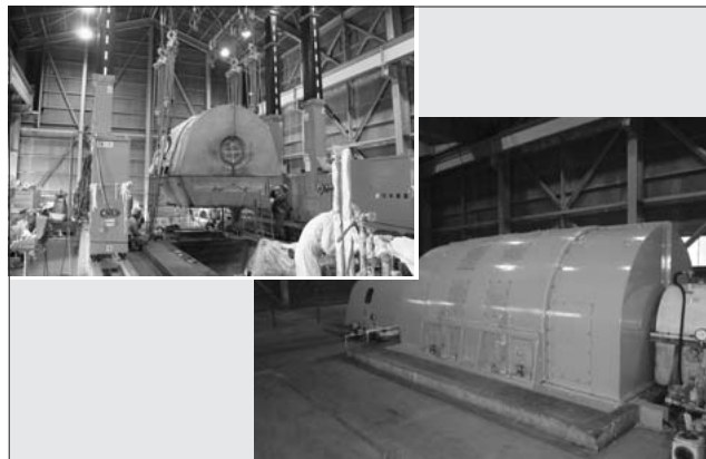
Fig.41 Transferring out of the former power generator stator and installation of the new power generator stator
