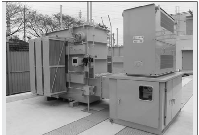
Fig.27 66 kV power-receiving and direct-current transforming facility
