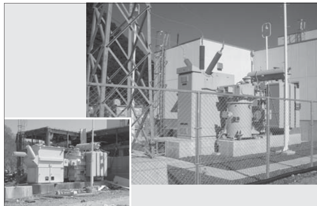
Fig.52 66 kV receiving and distribution facility immediately after disaster and after restoration
