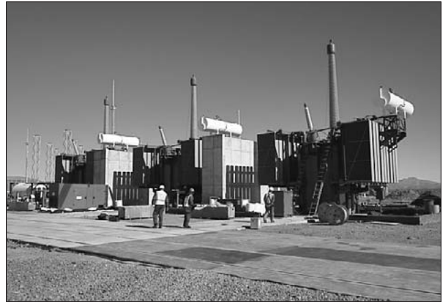
Fig.25 765 kV, 400 Mvar shunt reactor
