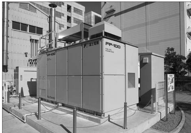
Fig.7 Fuel cell equipment installed in Kawasaki factory
