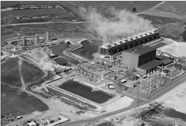
Fig.8 Overview of the Nga Awa Purua Geothermal Power Station
