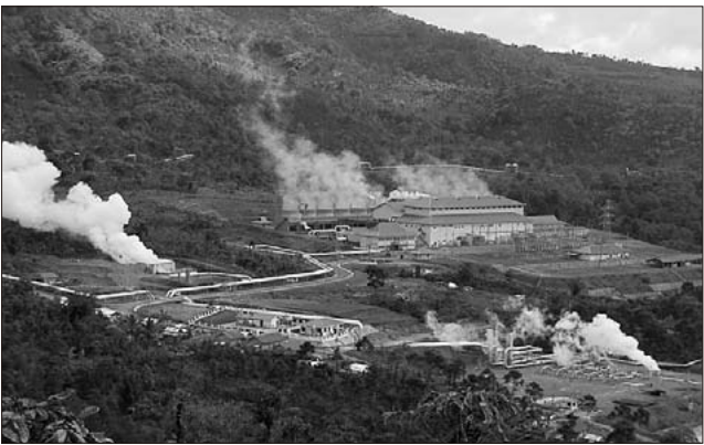
Fig.7 Panoramic view of Ulubelu Geothermal Power Station
