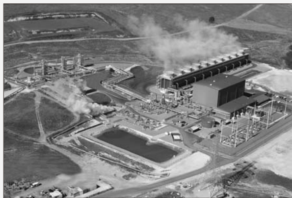
Fig.5 Nga Awa Purua Geothermal Power Station in New Zealand
