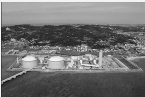
Fig.4 Yoshinoura Thermal Power Station of the Okinawa Electric Power Company, Incorporated (Photo: provided by the Okinawa Electric Power Company, Incorporated)
