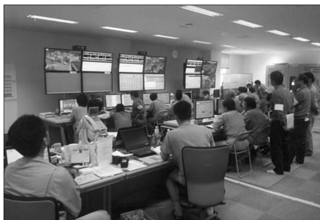
Fig.3 Central control room during load rejection tests
