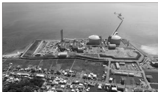
Fig.1 Panoramic view of the Yoshinoura Thermal Power Station
