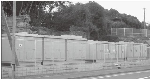
Fig.4 Storage system for 300 kW
