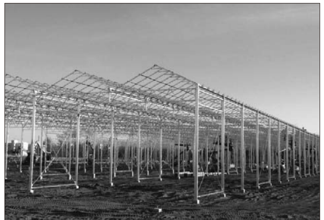
Fig.18 Greenhouse horticulture (under construction)
