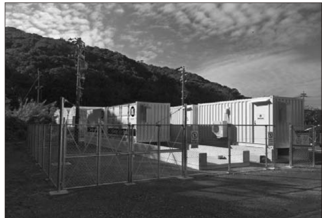
Fig.2 External appearance of Koshiki-shima Power Management Center
