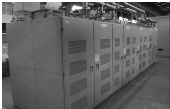
Fig.4 Large-capacity self-commutated flicker compensator for steelmaking
