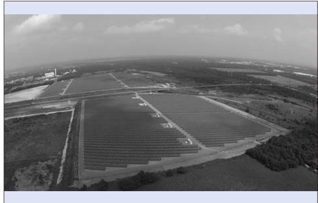
Fig.6 Full view of areas A and B in Tomakomai Yufutsu Mega-Solar Power Plant
