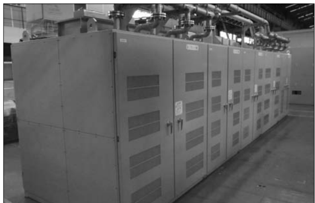
Fig.4 Large-capacity self-commutated flicker compensator for steelmaking
