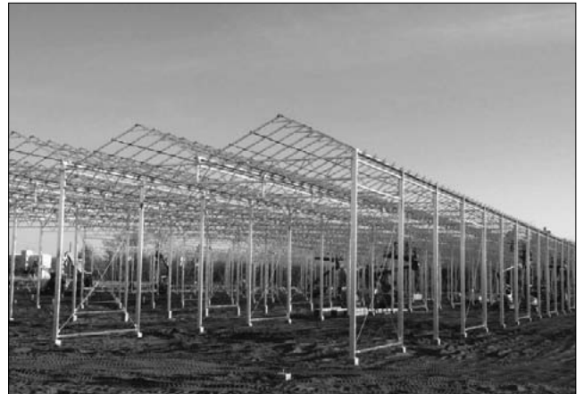
Fig.18 Greenhouse horticulture (under construction)
