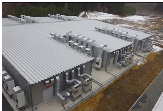
Fig.11 External appearance of module-type data center delivered to IDC Frontier Inc.
