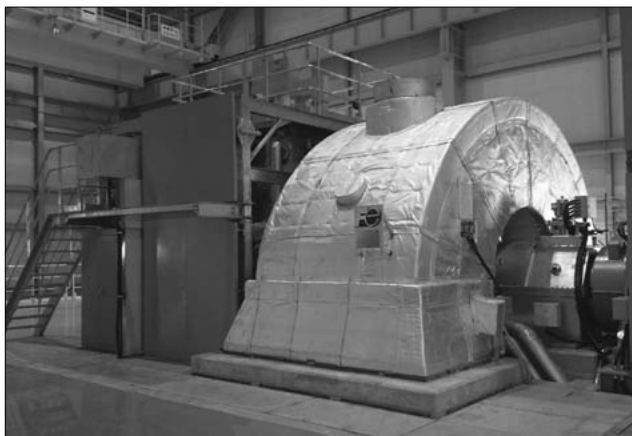
Fig.2 Reheat steam turbine
