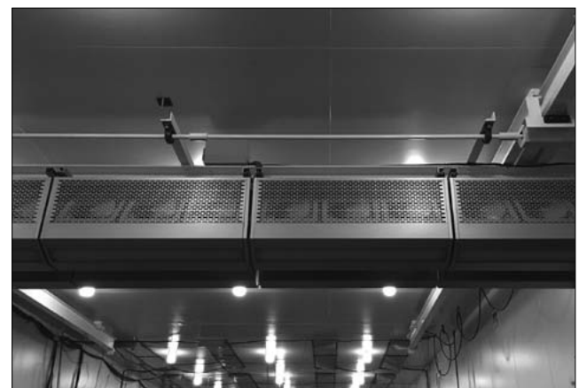
Fig.21 Zoning air curtain with moving mechanism
